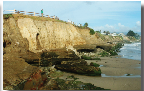
After stabilization and application of sculpted and stained shotcrete facing
